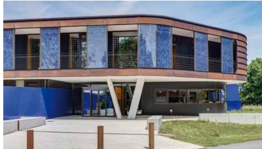
Photo: Office building | Eitting | Materials with patina - corten steel in combination with Photovoltaic panels | ArchitekturWerkstatt Vallentin GmbH | Germany © Photo: Jakob Kanzleiter
