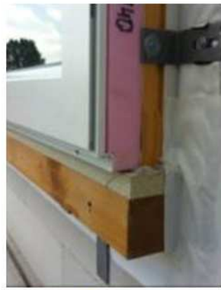
Finestra triplo vetro U_w = 0,74 \text{ W}/(\text{m}^2\text{K})
