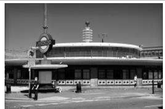
Southgate, Enfield's Art Deco London Underground station,
