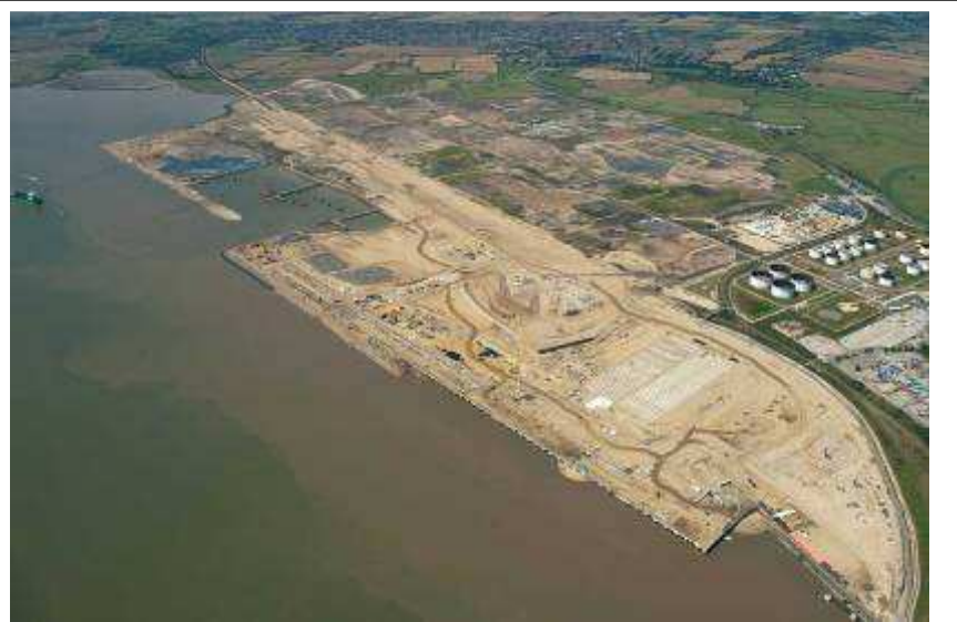
London Gateway port construction site, http://www.londongateway.com/
