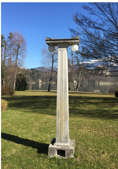
Figure 6: new luminaires on existing poles (Park Vila Bled)
